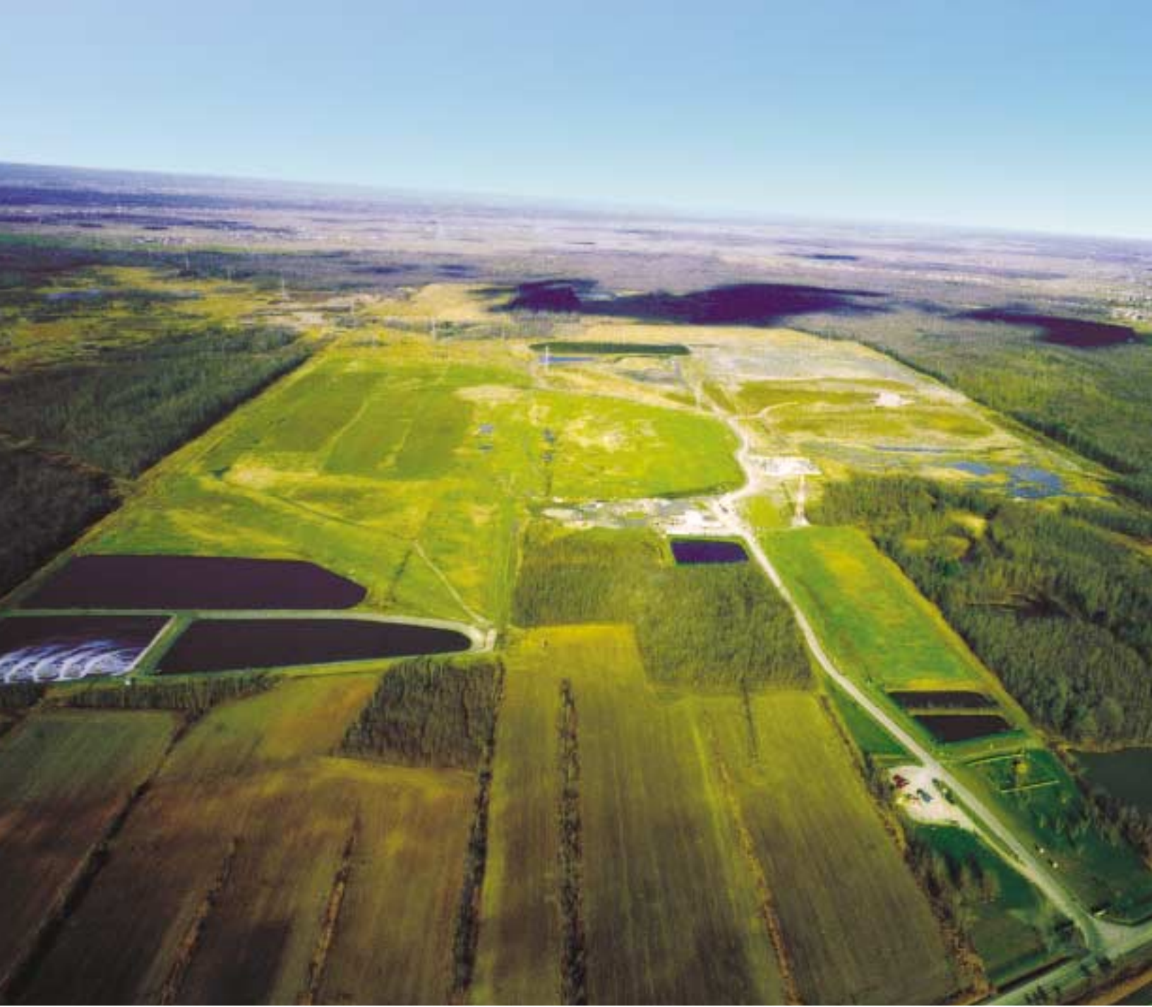
^ An aerial view of the Lachenaie landfill
